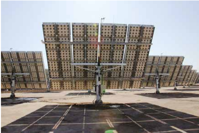
Picture 1: 200-kW CPV modules on a dual-axis tracker in Qingdao, China
