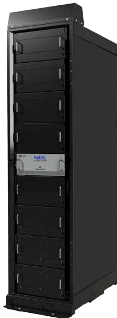
Picture 2: A High Rate (HR) Energy Storage Rack
