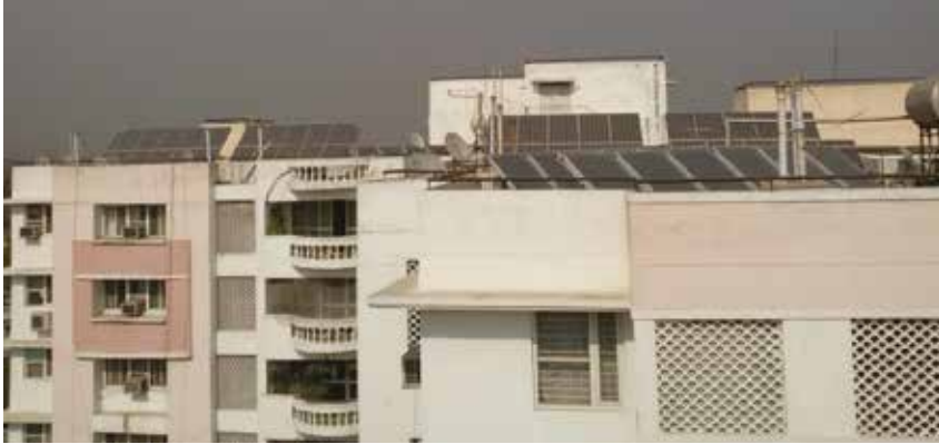
Picture 4: Solar PV array for lighting system installed in Type VI towers
