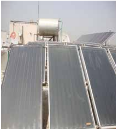
Picture 2: Solar water heating system (Type VI flat)
